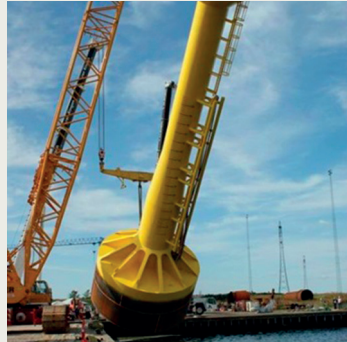
The bucket foundation is lowered into the water
