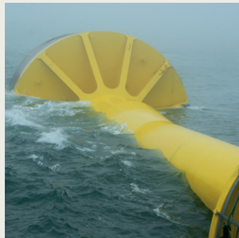
Bucket foundation being floated to site
