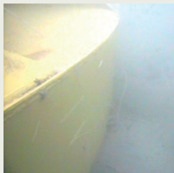
The bucket foundation during installation
