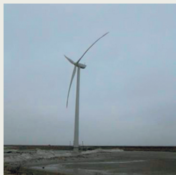
Successful completion of the project
