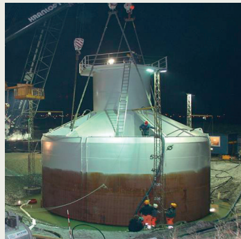
Bucket foundation being prepared for installation
