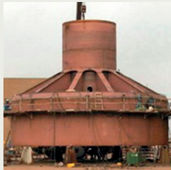
The bucket foundation during construction
